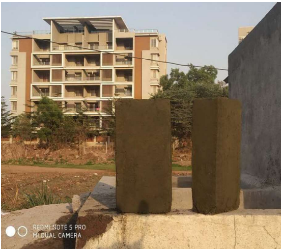
Fig No. 9 (Even surface obtained after plastering the columns casted using embossed plate formwork)
