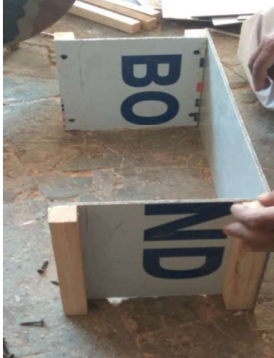
(Fig. Making of aluminum composite material mould for casting concrete block)
